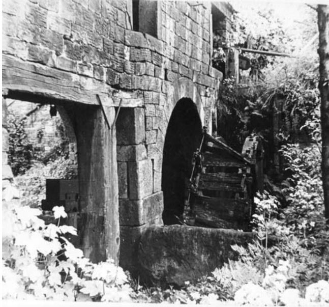
Figure 9 Derelict state of No.2 water wheel in the late 1950s. Note the wooden prop supporting the lintel and masonry of the Forge building. This was put in place as a short-term measure in 1955 by Oliver Inman who carried out emergency repair work. The prop could not be removed until 1975 after the structure had been consolidated.
