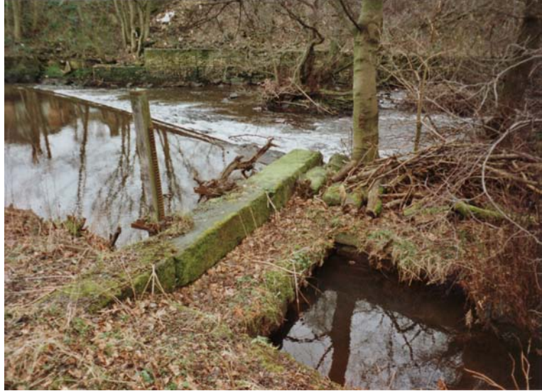
Figure 15 The weir, sluice gate and beginning of head goit
