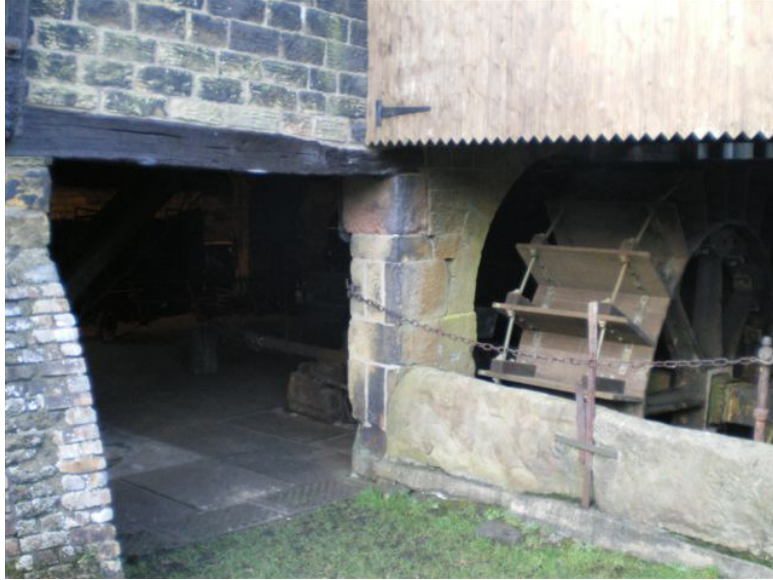
Figure 27 The restored No. 2 water wheel. The prop formerly supporting the lintel (see Figure 9) has been removed
